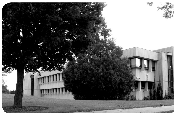
Central Michigan University's Foust Hall houses the Office of Research and Graduate Studies.
